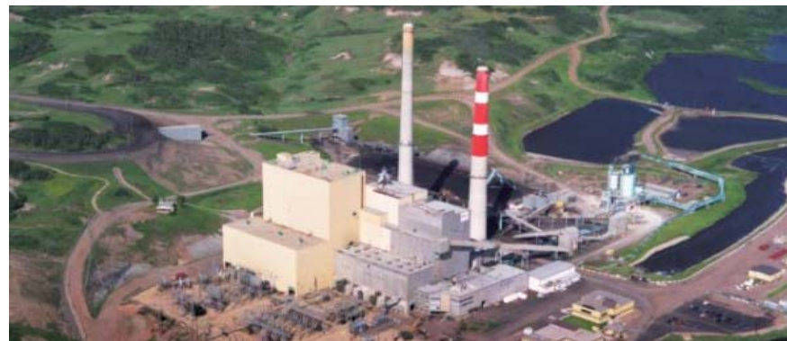
Battle River Generating Station
