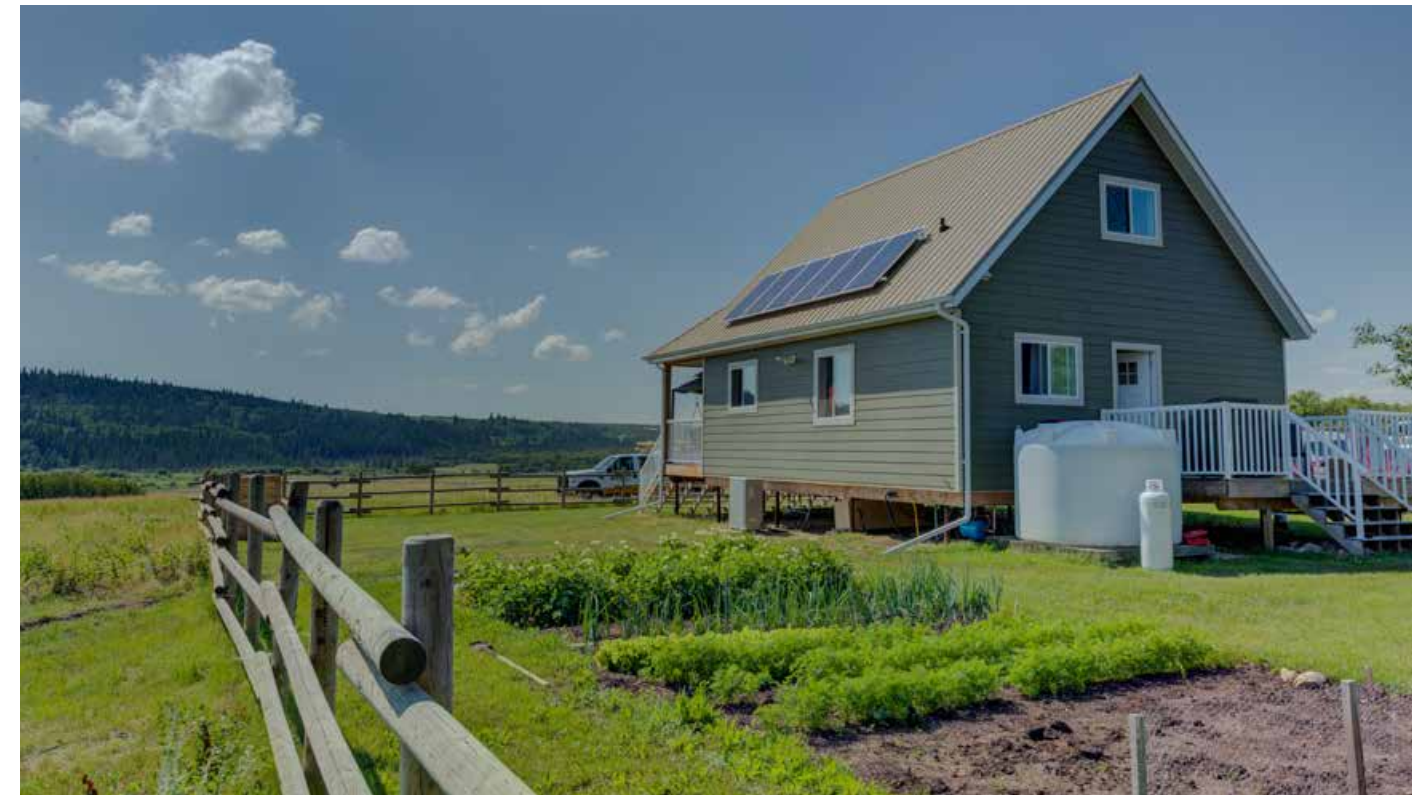
Our hybrid house project in Mannville, Alberta utilizes micro-combined heat and power, solar and battery storage.
